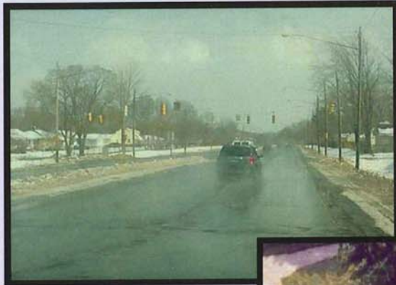
SR 57 before rehabilitation project
