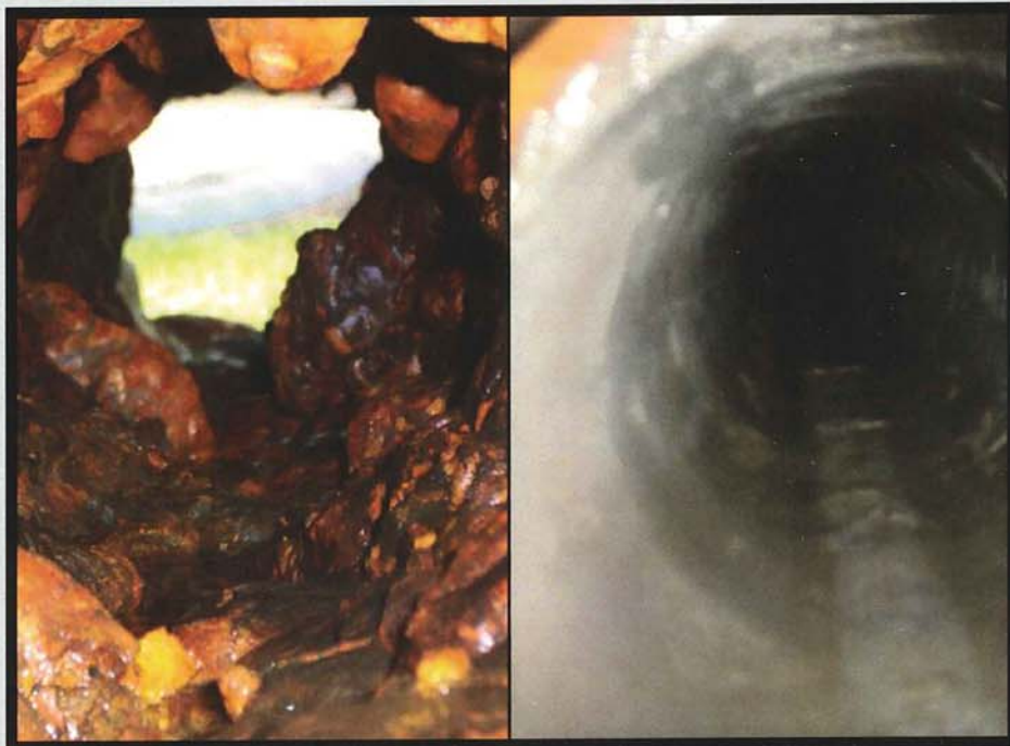
After water line cleaning project.
