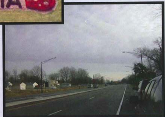
SR 57 after rehabilitation project
