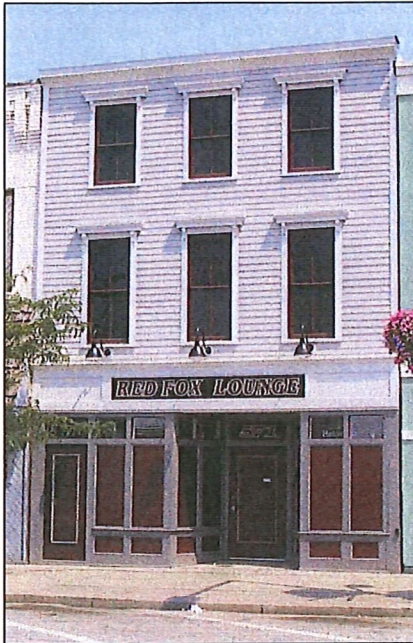
Restored wood facade
