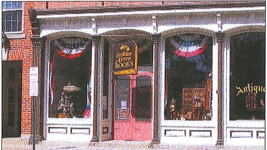
Storefront details of columns and brackets
