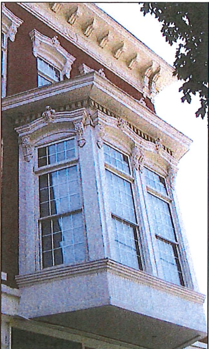
Bay window with complimenting cornice
