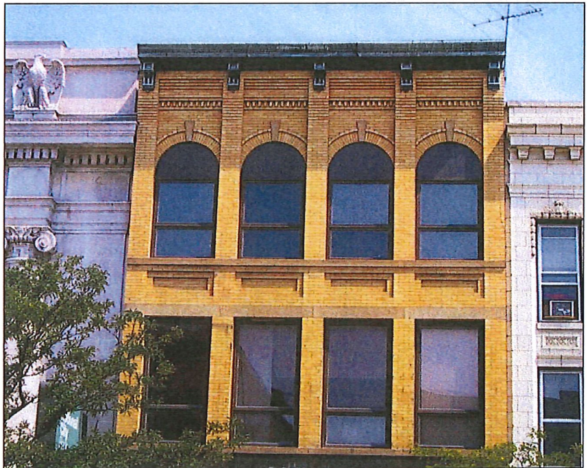
Metal and decorative brick cornice
