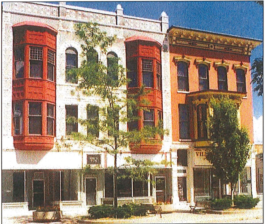
Painted masonry with historic color scheme
