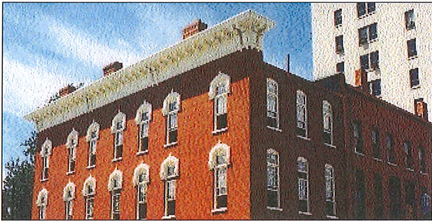
Cornice and parapet conceal sloped roof from main views
